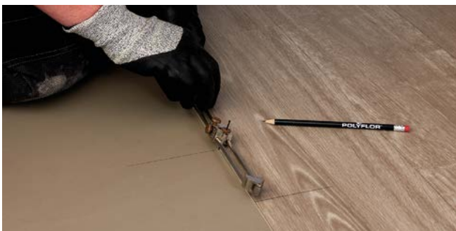
Figure 4 Scribing the wall profile
