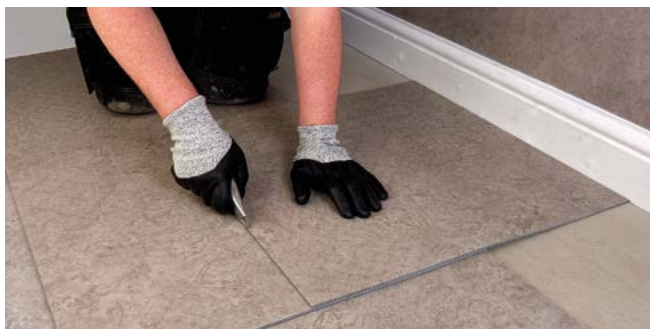
Figure 8 Measuring using an overlapping tile
