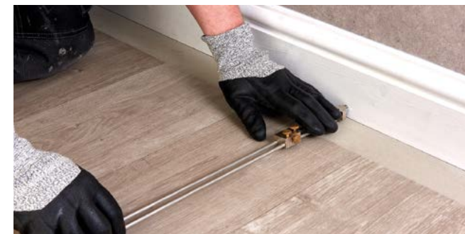
Figure 2 Scribing the wall profile
