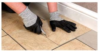
Figure 6 Measuring using an overlapping tile
