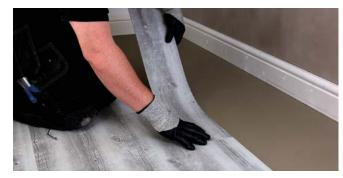
Figure 1 Setting planks out
