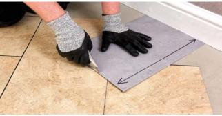
Figure 9 Cutting the perimeter tiles (diagonal cut)
