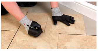
Figure 8 Marking using an overlapping template on diagonal laid tiles
