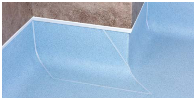
Figure 11 External corners 'wrap around method'
