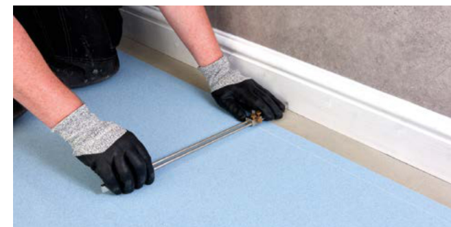
Figure 2 Scribing the wall profile
