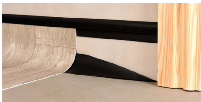
Figure 7 Taper towards a doorway
