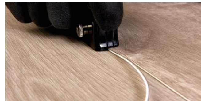
Figure 5 Cutting in the seams
